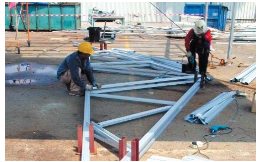
Install subsequent trusses over the truss template
